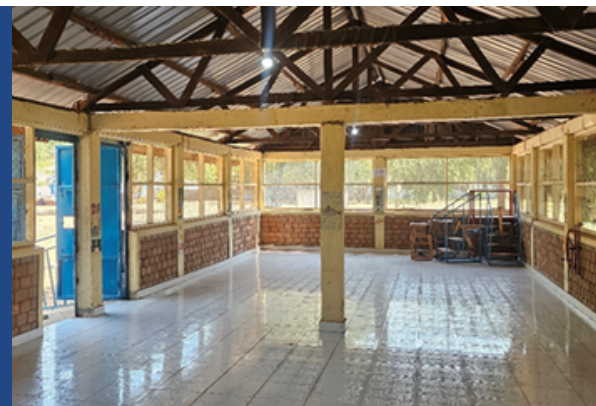
Empty Doro Day Care Center
